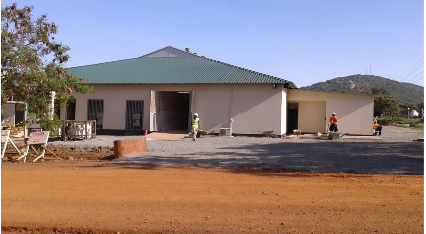
Photos of ongoing Construction of Mess at HME Geita Gold Mine.
