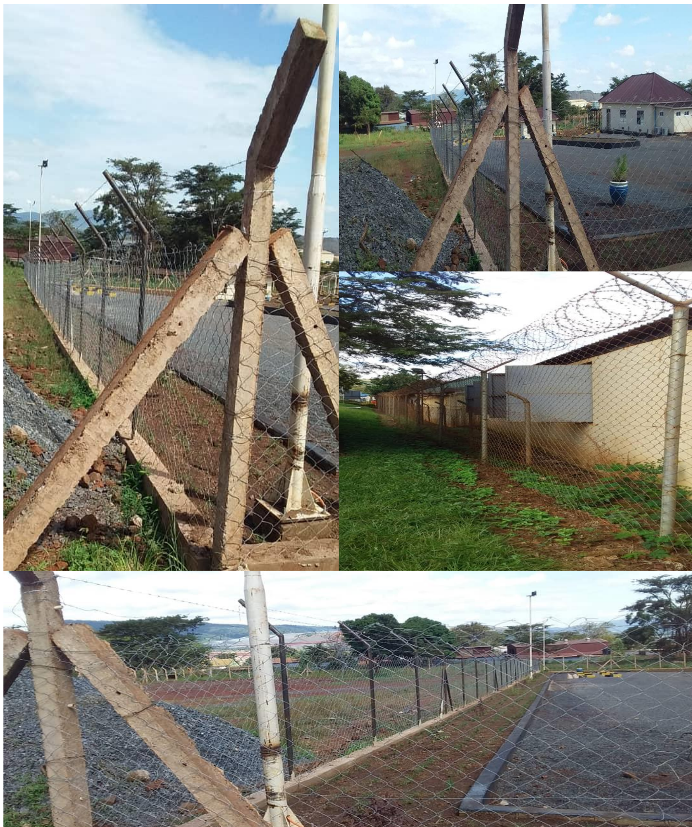
Photos of previous Installed Chain-link Fence at Geita Gold Mine.
